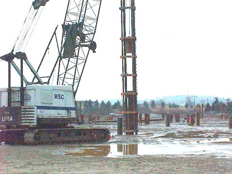
Drop hammer riding in front of leads driving concrete spun piles.
