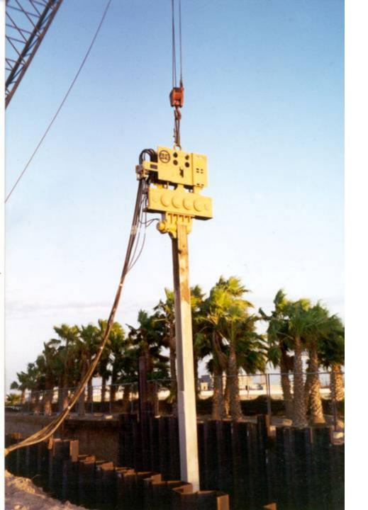
H-Beams being driven using an APE Model 200 vibro in Saudi Arabia
